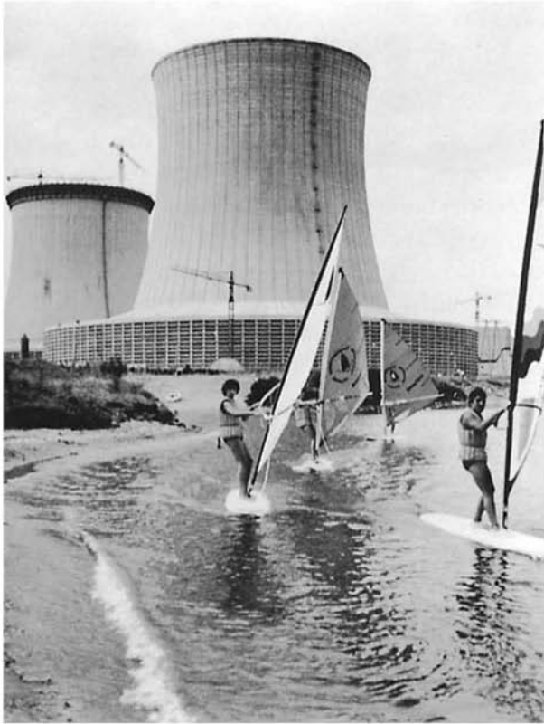
Windsurfers in front of the new cooling towers at the Saint-Laurent site in 1979. Source: EDF Photothèque.
